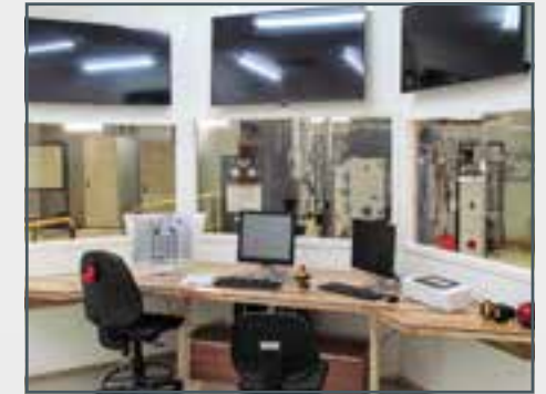
Module D control station
