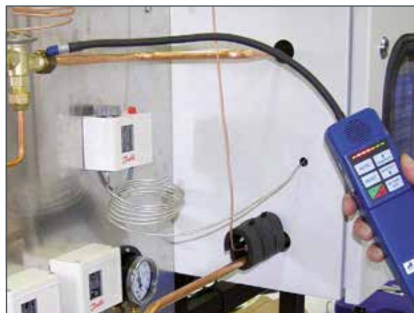
Leak testing at expansion valve
